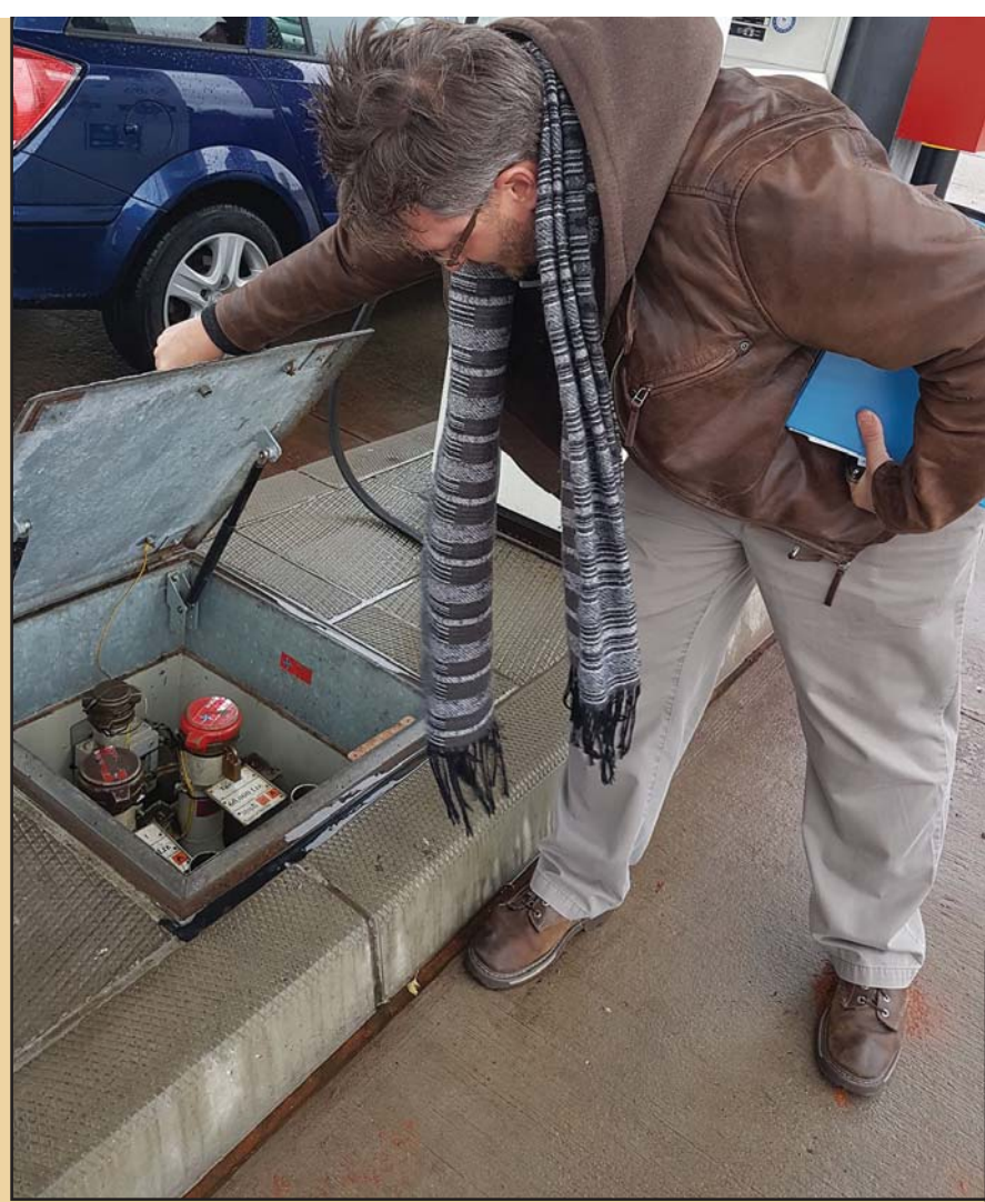
Resolution Specialist Keith Embree checks to make sure the tops of underground tanks are secure at Sembach Kaserne. Photo by Tawnya Moreno
